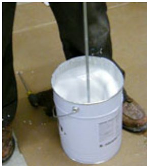
4. Mix for approx. 5 minutes. Use complete kit in the proportions supplied. (Do not alter proportions.)
