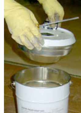
3. Completely drain Part B (hardener) into Part A (resin).
